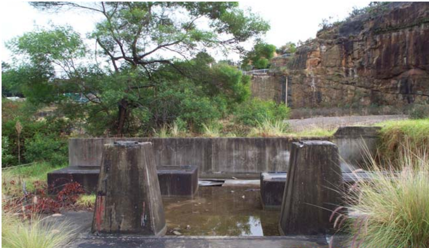
Remnant concrete blocks
