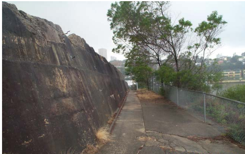
Current access – Site 1 to Site 3
