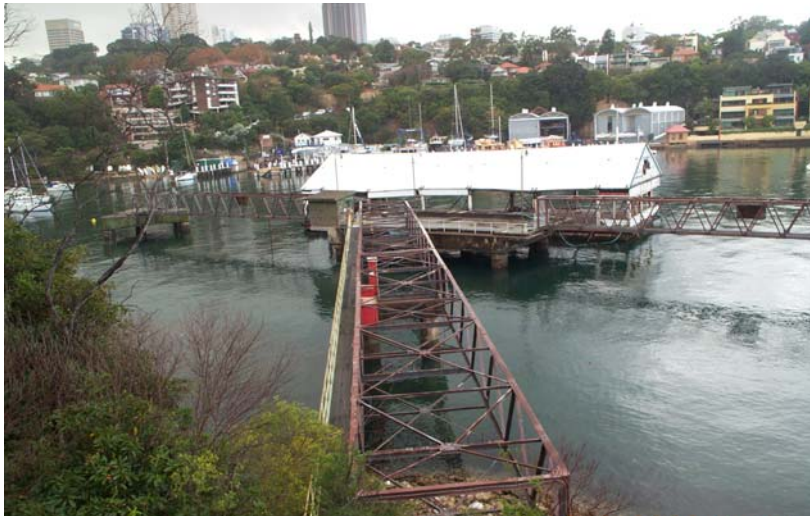
Site 3 – dolphin and access structures
