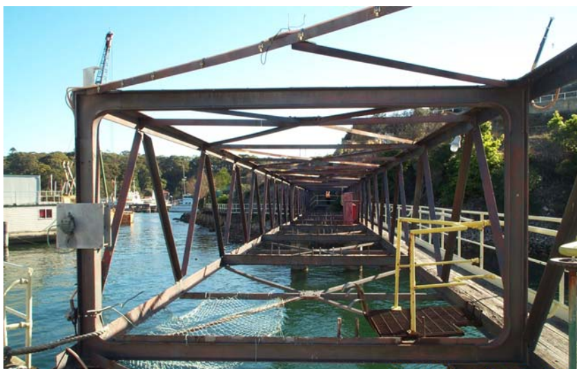
Site 3 - Pipe gantry support structure and access walkway
