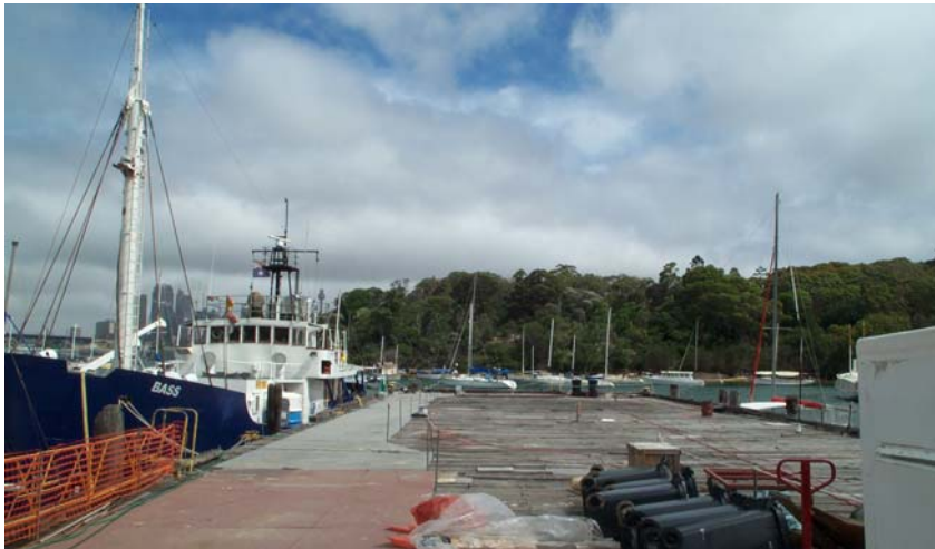
Wharf 1 on Site 1
