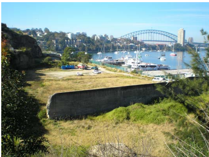
Stone wall facing eastward
